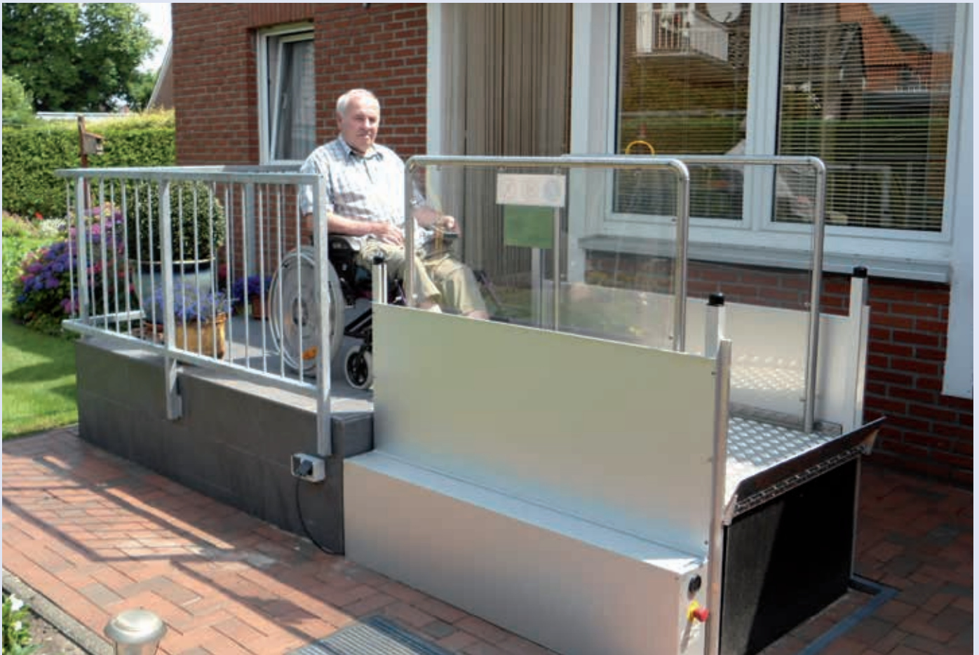
The terrace offered the best preconditions for the access route of the lifting device
